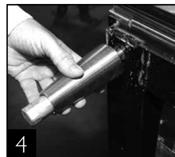
4 Thread leg into cabinet bottom frame rail.
